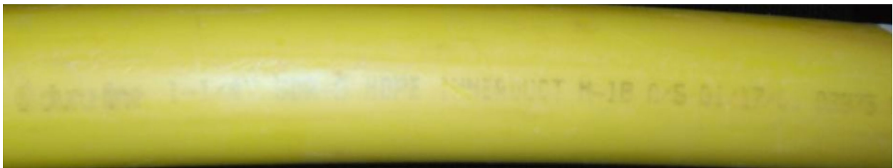
Figure 2: Print Line of Exhumed Conduit
